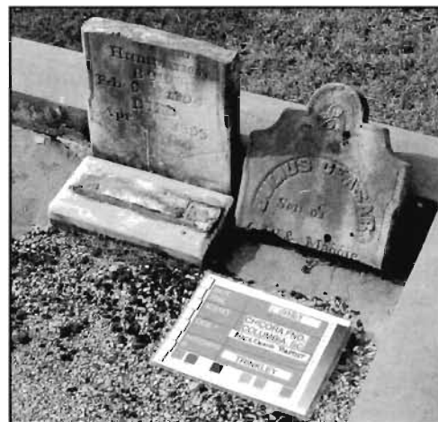
No matter how much epoxy is used, repairs like this are doomed to failure—and can often result in additional damage to the stone as the epoxy joint fails.
